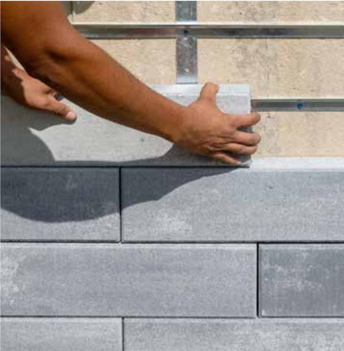
The U-Cara Wall Mount System allows you to put the finishing touches on your project by cladding existing structures like unsightly exposed foundation areas or concrete steps with U-Cara fascia panels.
